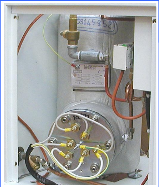
CALDAIA CHAUDIERE BOILER
